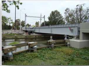
ST. ANN BRIDGE - SWING SPAN
