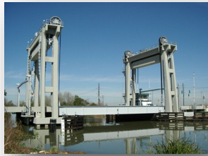
BAYOU LAFOURCHE BRIDGE
