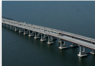
I-10 TWIN SPAN BRIDGE
