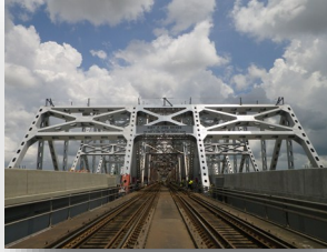
HEUY P. LONG BRIDGE
